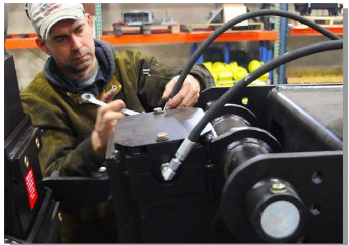
#18) Connect all hydraulic hoses. Hoses are labeled for easy installation. Cycle the Zacklift to expel air from system.
